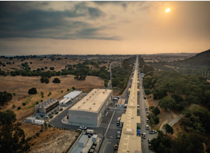
The LCLS-II cryoplant, which takes liquid helium from white tanks (in the middle left) via a transfer line (middle) to the superconducting niobium cavities, housed inside cryomodules within the accelerator tunnel (beneath the long narrow building running from bottom to top).
